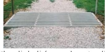
pickups to tractor trailers. The open rail cattle guard is placed in fence gaps where a gate would normally be installed to allow for easy vehicle or pedestrian access while keeping the livestock
